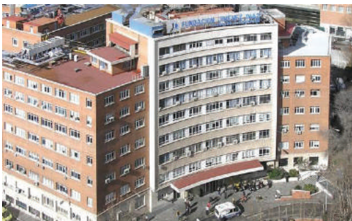
Hospital fundacion jimenez Diaz (Madrid )
